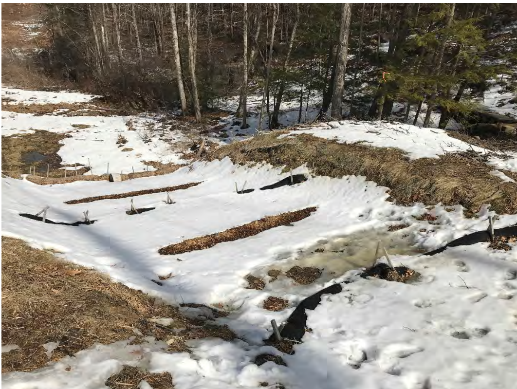
Fig 8: Lower portion of slope between Strs. 28 and 29. Viewing northeast. (03-10-21)
