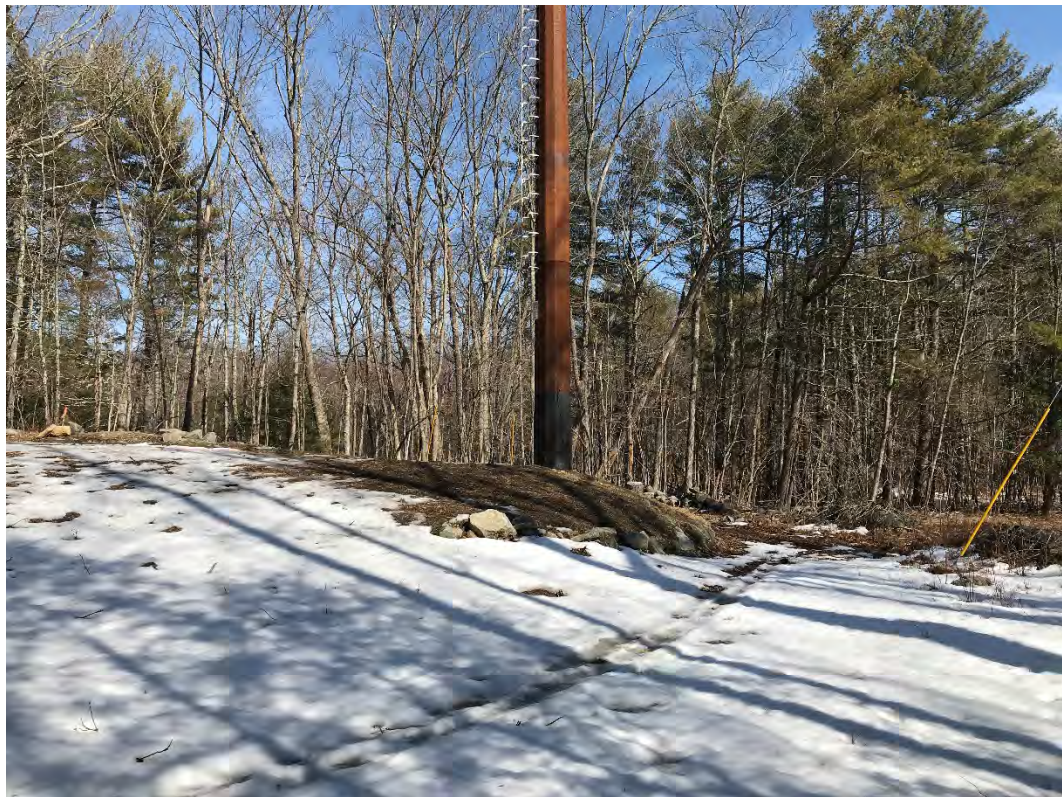
Fig 6: Str. 90 work area. Viewing northeast. (03-10-21)
