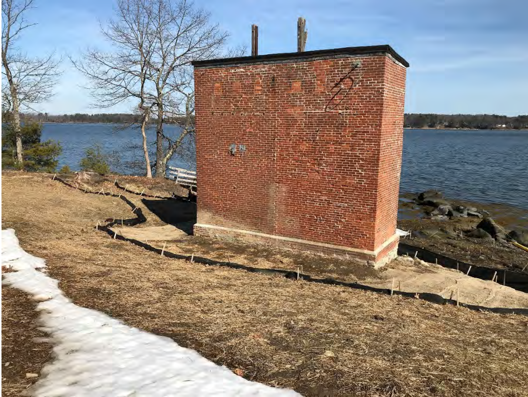
Fig 1: Slope leading down to cable house and salt marsh restoration at the Eversource property/west side of the bay. Viewing northeast. (03-10-21)
